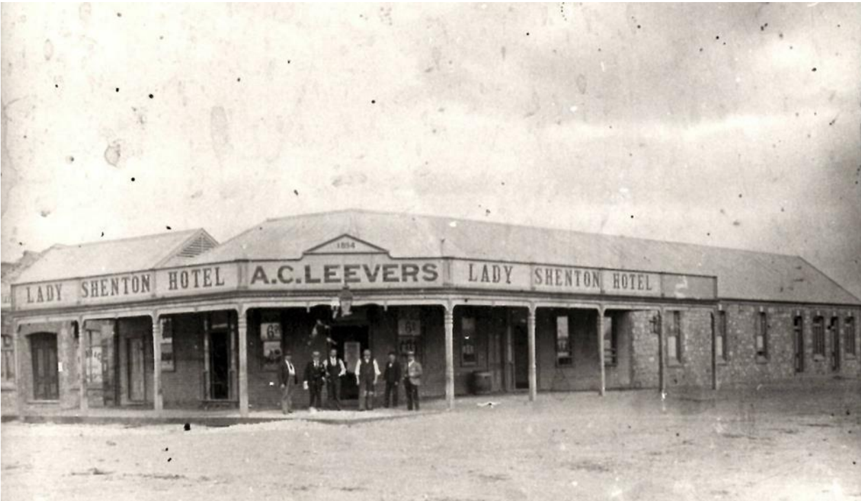
Figure 4: Lady Shenton original centrally Pitched Roof
