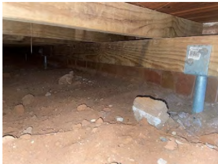
Plate 43 – Re-stumping to back extension using proprietary stirrups
