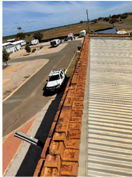
Plate 53- Parapet with capping brick
