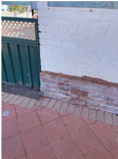
Plate 1 – Cement Render removed from lower pedestal
