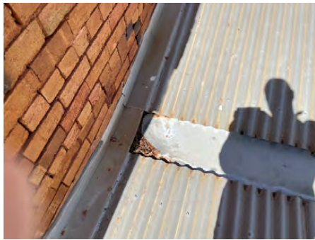
Plate 47 – Start of shallow box gutter
