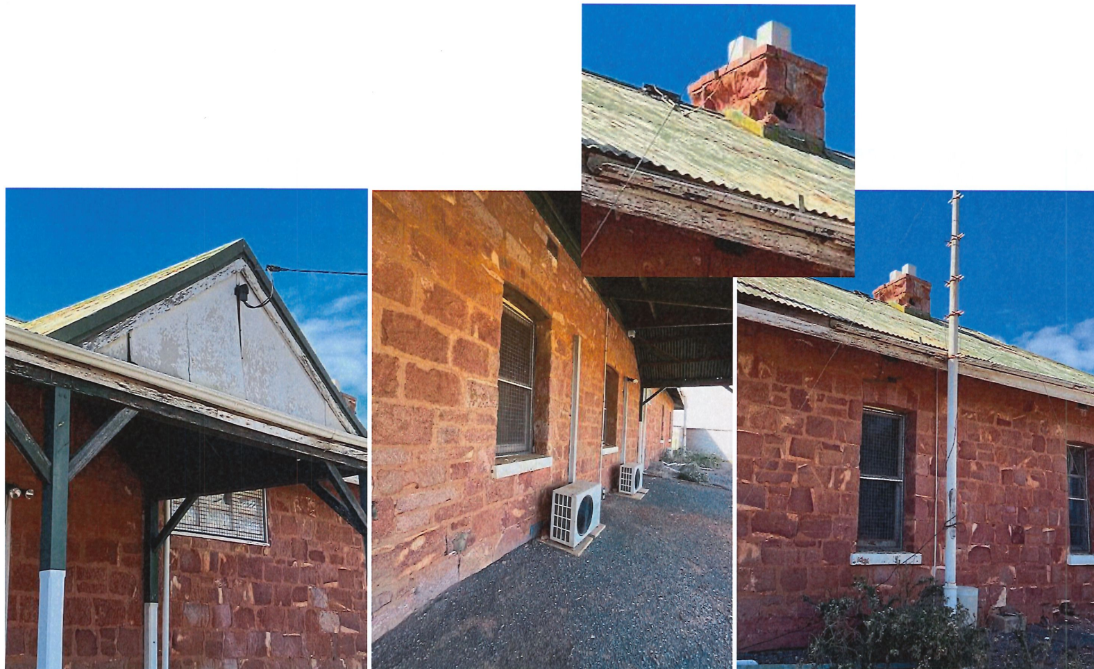
Photos 12, 13, 14, 15 View south across the west frontage towards the south end showing the deteriorated timbers and gable infill, missing gutters, and seriously eroded stone chimney with inadequate flashings.
