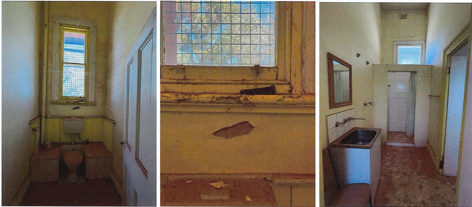
Photos 50, 51, 52 Interior: Ladies room toilet and detail of timber and wall damage (west wall), and laundry and shower (east end).
