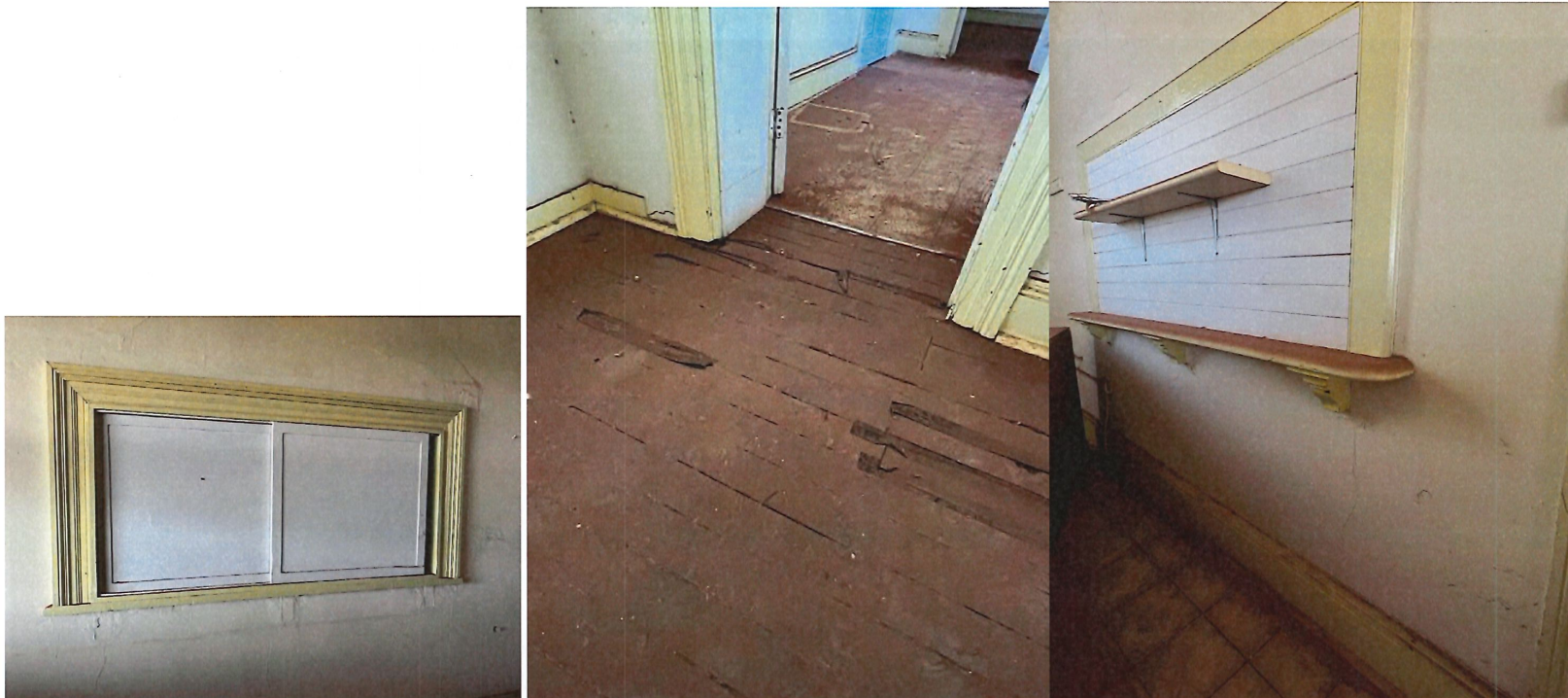
Photos 73, 74, 75 Interior: Refreshment room showing servery on south wall, timber floor damage at doorway through to the kitchen, kitchen side of the servery.
