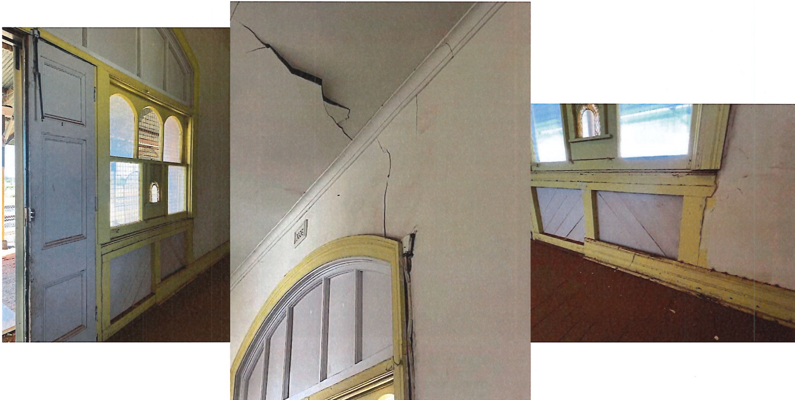
Photos 60, 61, 62 Interior: Luggage room showing arched window set, damage to wall and ceiling and at dado level.
