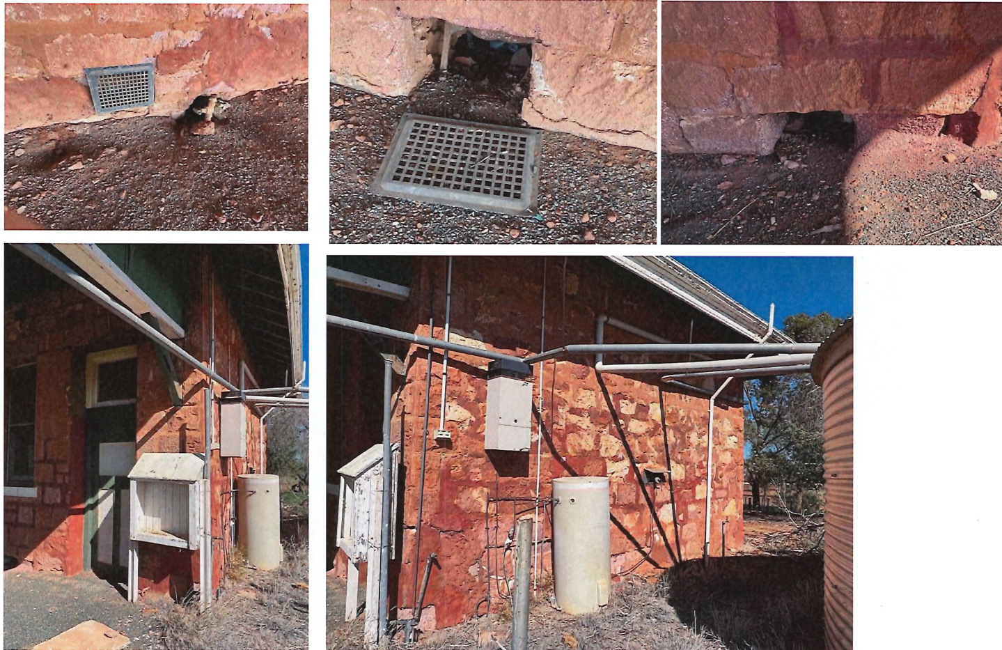
Photos 39, 40, 41 Examples of vents and vent openings along the base of the platform wall.
