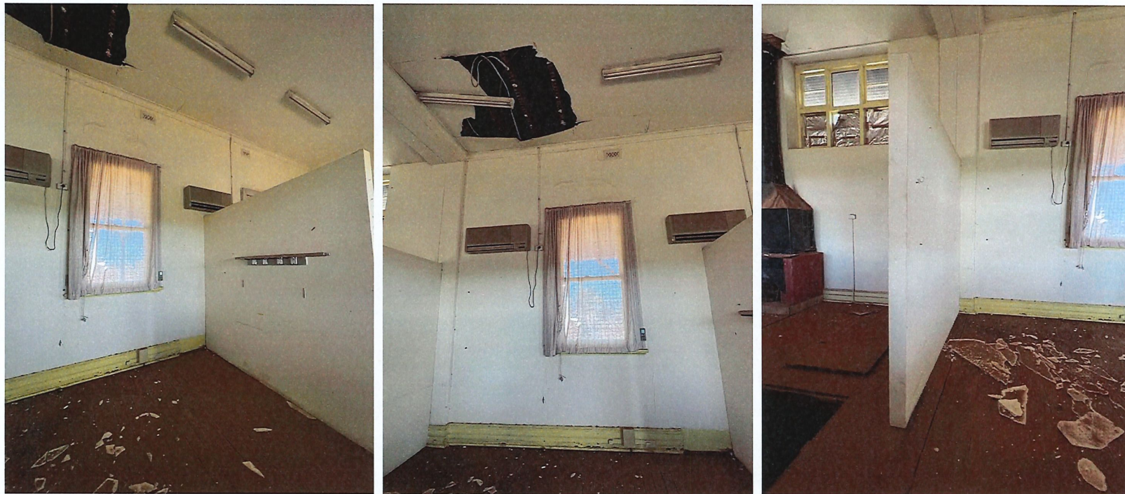
Photos 63, 64, 65 Interior: Luggage room showing timber framed partiitons and ceiling damage. The second partition is where the original wall between the luggage room and refreshment room was located.
