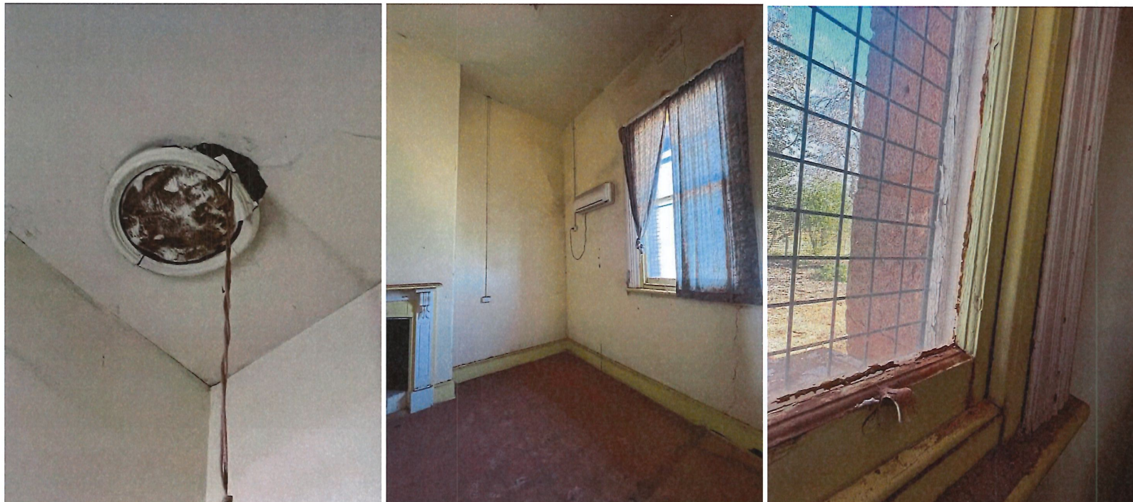
Photos 47, 48, 49 Interior: Ladies room partitioned section on the west side- damaged ceiling vent, west frontage window, and window frame detail.
