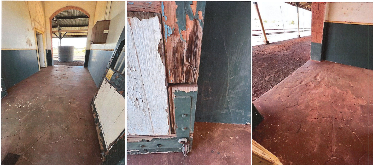
Photos 19, 20, 21 View of the luggage entrance looking to the east, showing the concrete floor, damaged gate that evidences previous interventions, and detail of the concrete floor.
