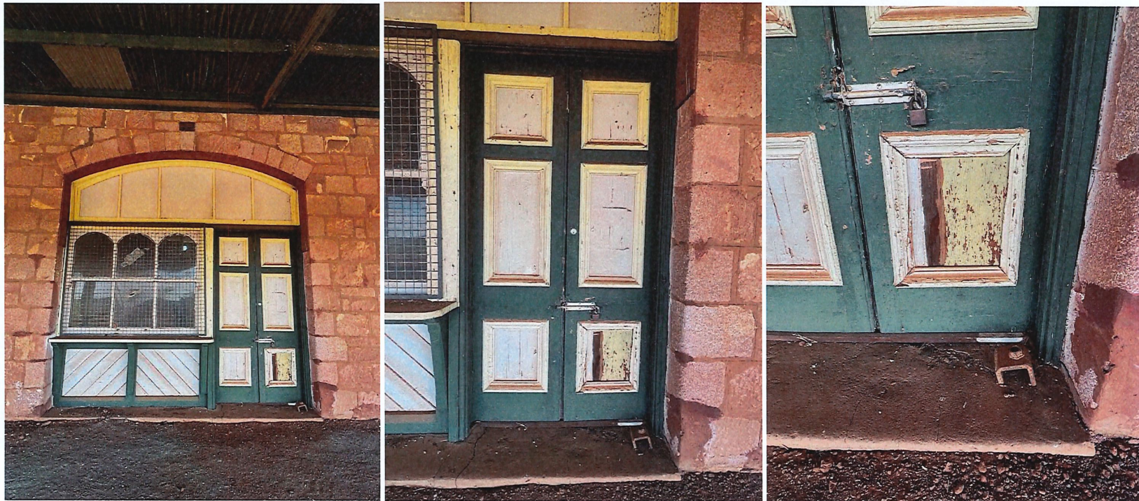
Photos 29, 30, 31 The arched window set and pair of paneled entry doors into what was the refreshment room off the railway platform, showing timber damage and deterioration.
