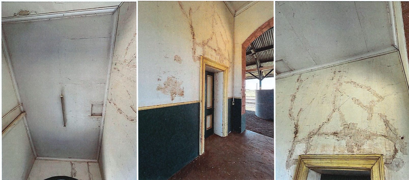
Photos 22, 23, 24 Views in the luggage entrance showing the ceiling, door to the ticket office and detail of the wall condition above that door.
