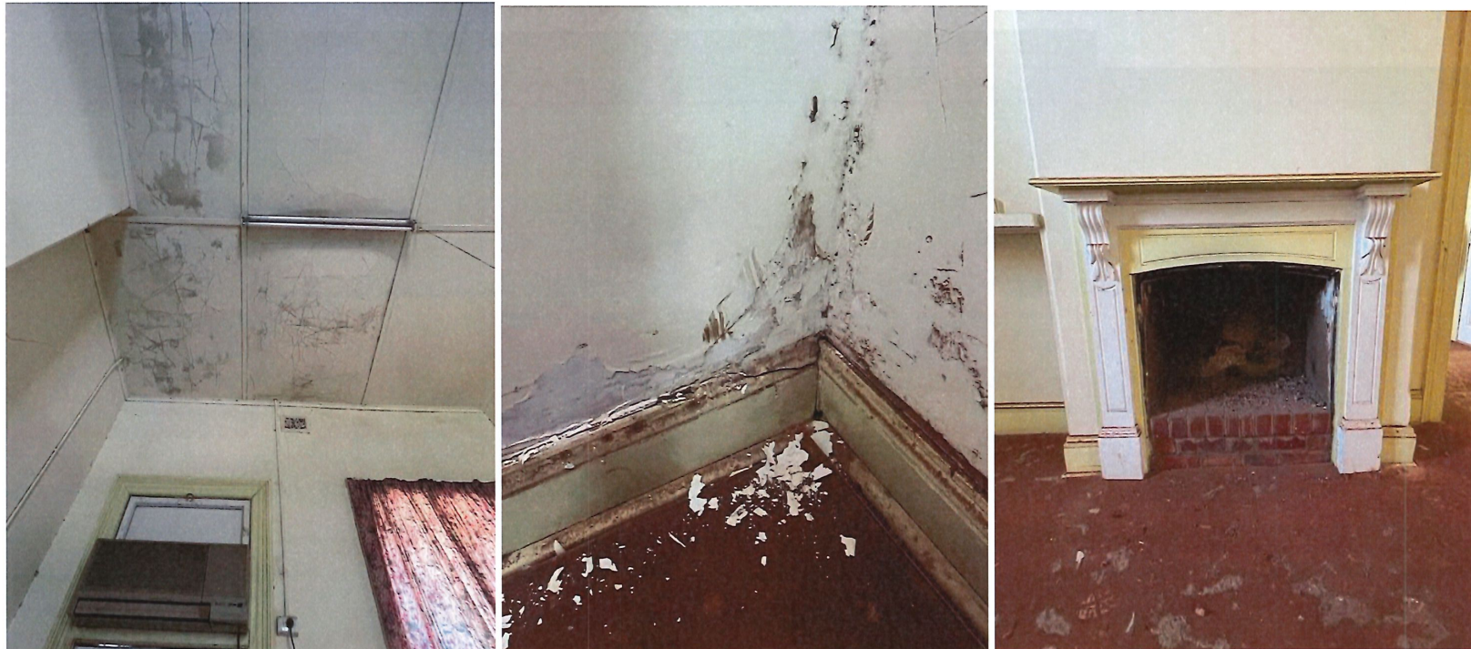
Photos 80, 81, 82, 83 Interior: Stationmaster's room showing moisture damage to the ceiling in the northwest corner, moisture damage on the lower wall in the southeast corner, and the intact fireplace on the north wall.
