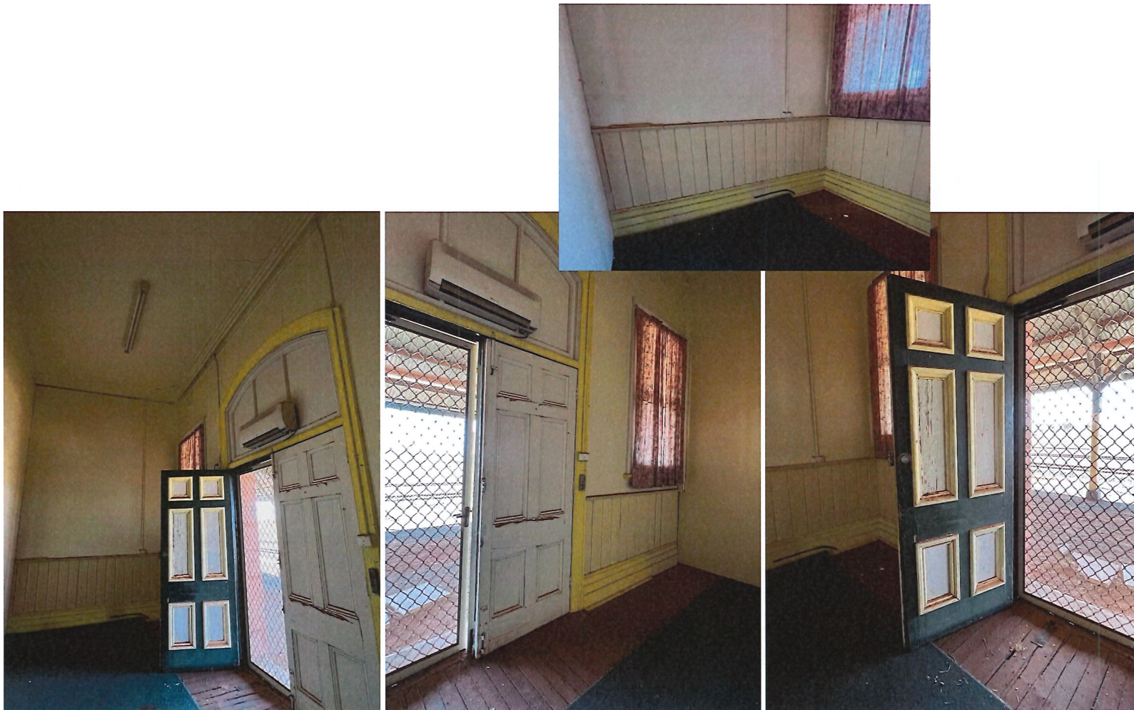
Photos 53, 54, 55, 56 Interior: entry off the platform into waiting room showing partition on the west side (left); doors detail and floor damage. Inset- dado detail.
