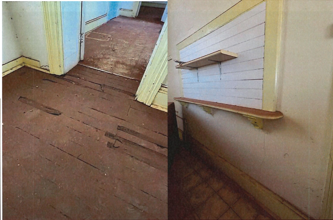
Photos 73, 74, 75 Interior: Refreshment room showing servery on south wall, timber floor damage at doorway through to the kitchen, kitchen side of the servery.
