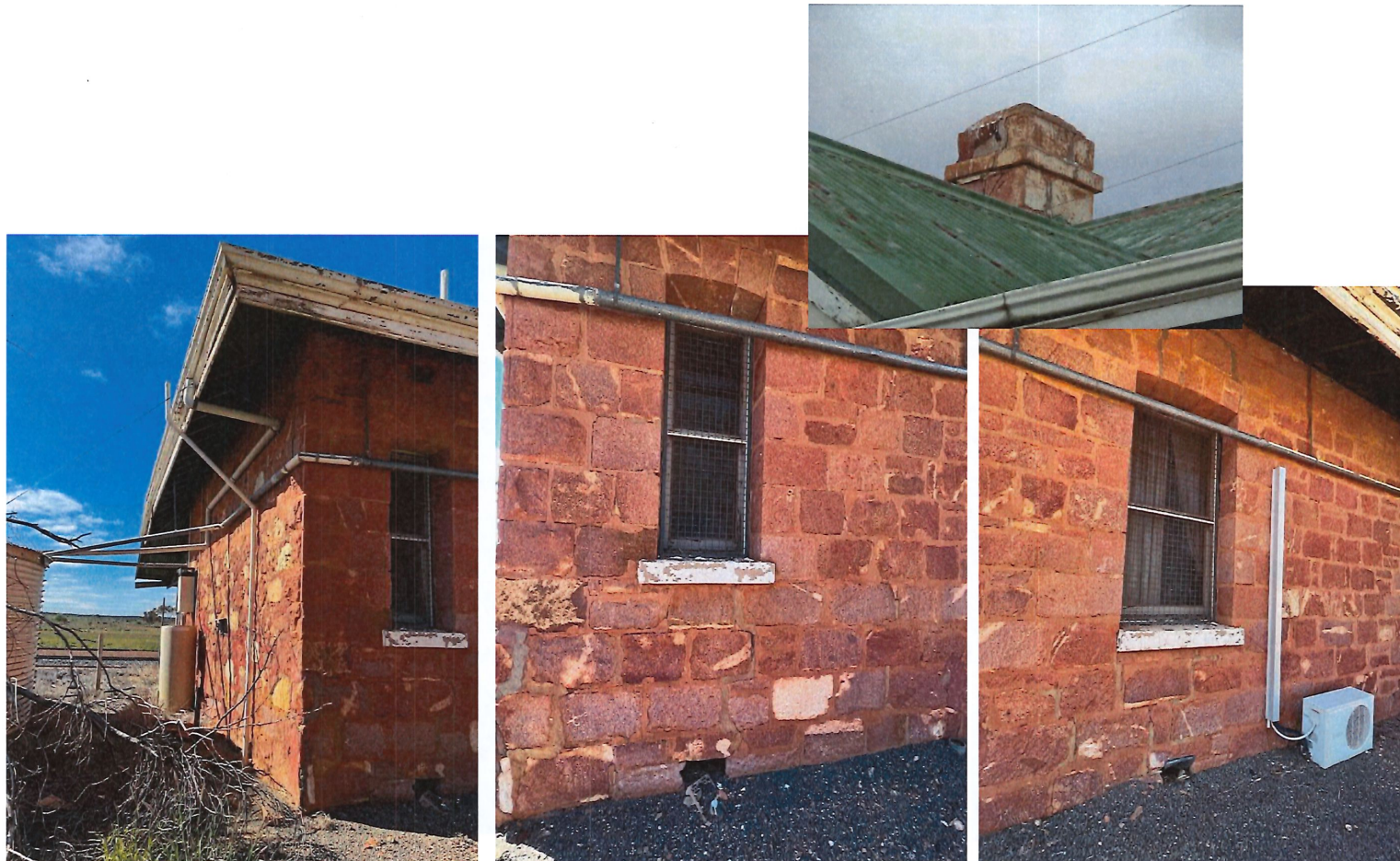
Photos 4, 5, 6, 7 The north end of the west frontage showing the face stone, airvent openings, weathered timber details, pipes from the gutters to the rainwater tank, and split system airconditioners. Inset above: north end chimney.
