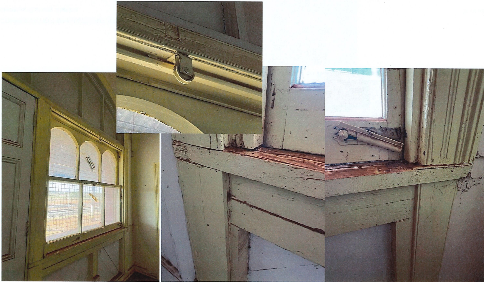
Photos 69, 70, 71, 72 Interior: Refreshment room showing arched window set, pulley detail, and hardware and timber detailing.
