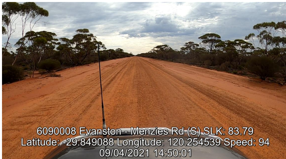
Post Damage Photo (After Photo 38)
