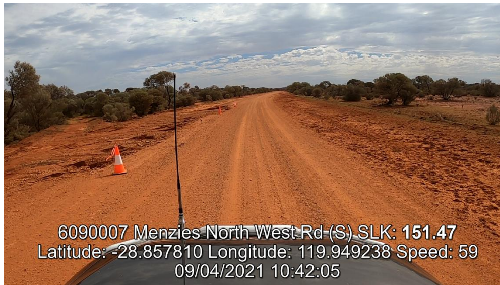
Post Damage Photo (After Photo 349)
