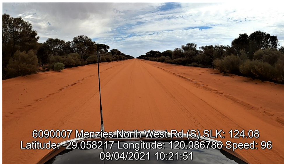
Post Damage Photo (After Photo 258)
