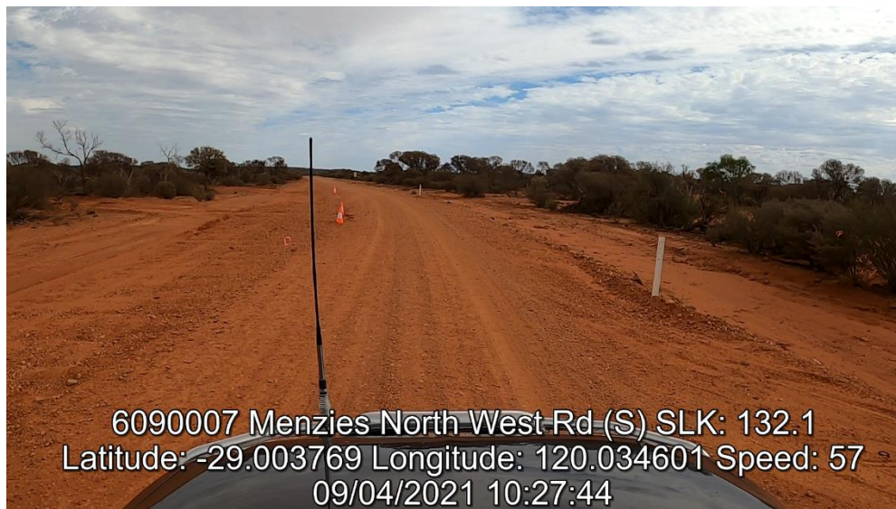
Post Damage Photo (After Photo 285)
