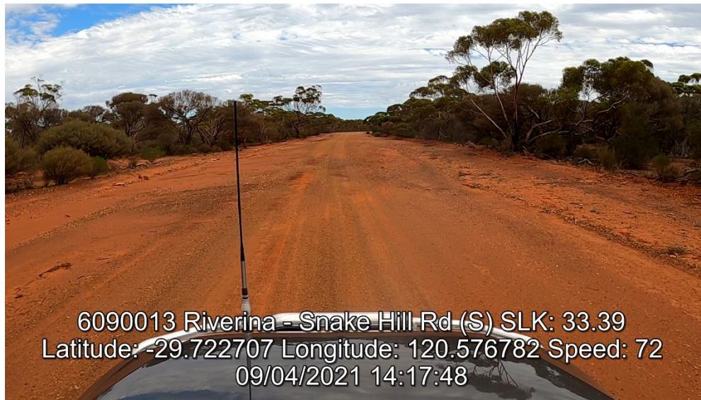
Post Damage Photo (After Photo 76)
