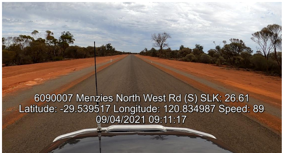
Post Damage Photo (After, Photo 68)
