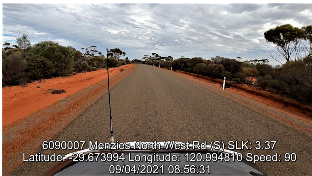
Post Damage Photo (After, Photo 4)
