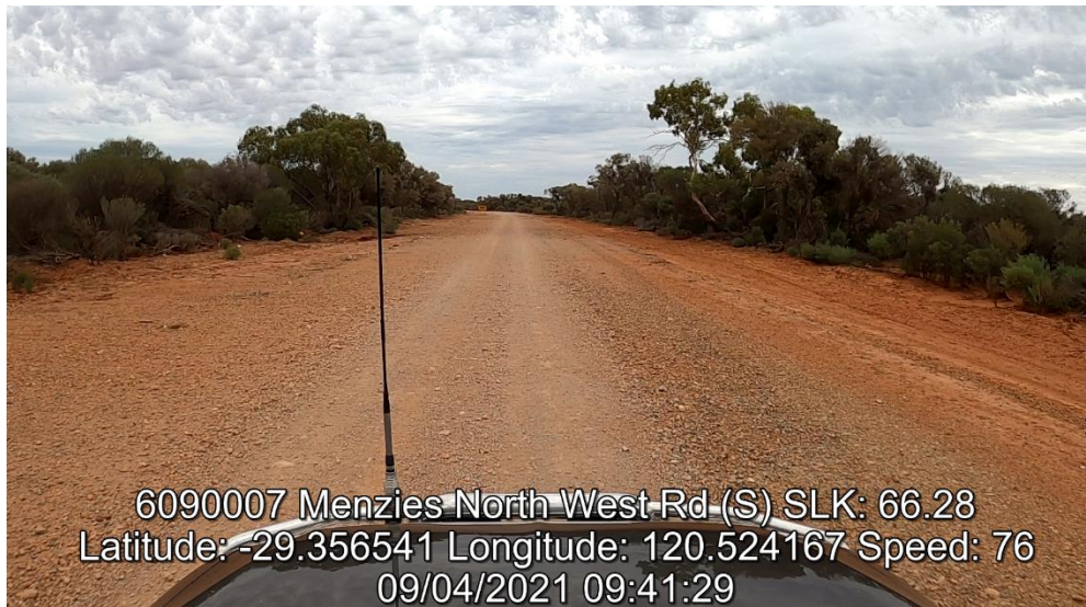
Post Damage Photo (After Photo 165)
