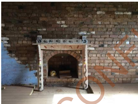
Photo 31 -Detail view of timber mantelpiece and fireplace in Old Tearooms & Butcher Shop.
