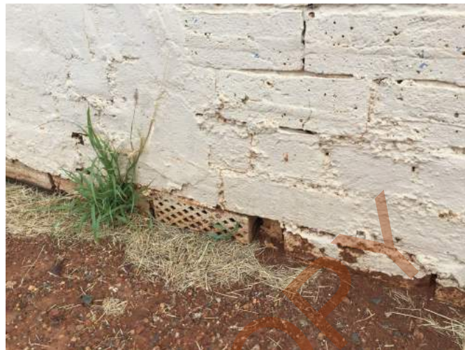
Photo 16 - Detail view of original sub-floor vent that has been compromised by concrete floor slab and raised ground levels
