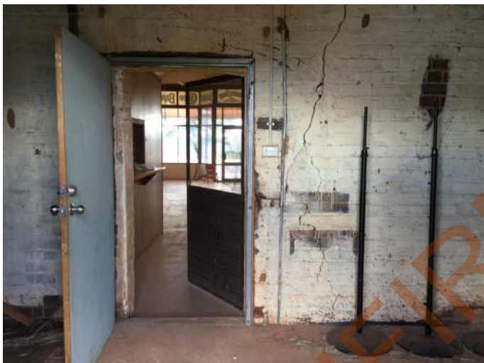
Photo 13 - Interior view from rear lean-to addition looking west into Old Pioneer Store. Note the structural cracking through the masonry
