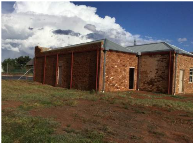
Photo 24 - North and rear elevation of Old Tearooms & Butcher Shop showing recent stabilisation works and new roofing.
