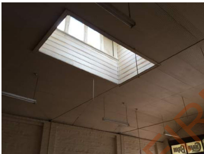
Photo 9 - Detail view of roof lantern located centrally in ceiling. Note also the canted ceiling shape which is lined with mini-corrugated iron
