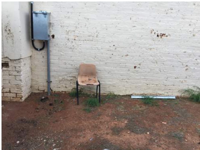
Photo 15 - Detail view of new electrical services mounted on south wall of Old Pioneer Store
