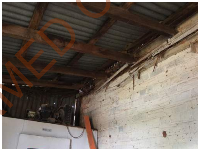
Photo 14 - Detail view of termite damage to timbers in lean-to addition to rear of Old Pioneer Store
