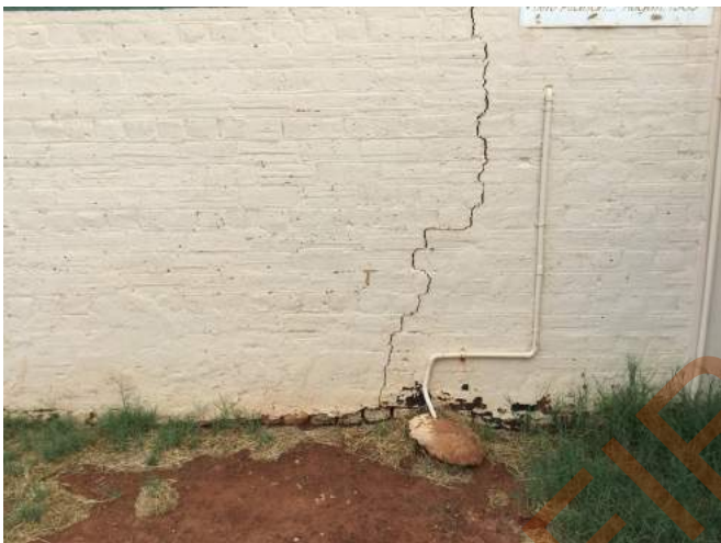
Photo 17 - Detail view of structural cracking evident in external walls of Old Pioneer Store
