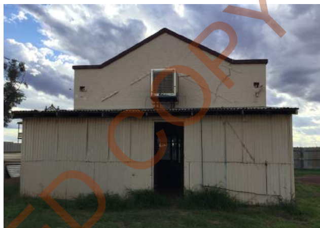
Photo 2 - Rear elevation of Old Pioneer Store showing existing lean-to addition and evidence of line of old gable roof to parapet wall.
