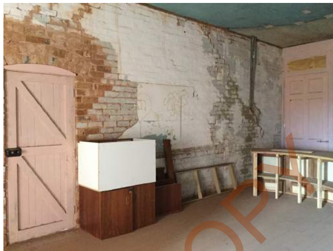
Photo 30 -Interior view of northern tenancy of Old Tearooms & Butcher Shop showing old countertop and lined & ledged door
