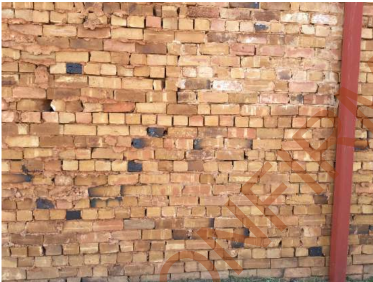
Photo 27 -Detail view of colonial bond brickwork, showing areas where re-pointing is required
