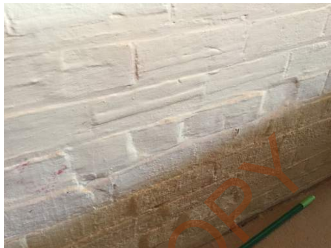
Photo 12 - Detail view of evidence of rising damp to interior walls of Old Pioneer Store
