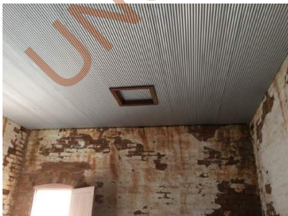
Photo 33 - Detail view of typical masonry walls and replacement ceiling to section of Old Tearooms & Butcher Shop
