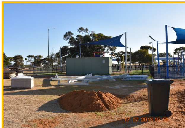
The shade structure lays on the ground awaiting the crane to move it into position over the outdoor area.
